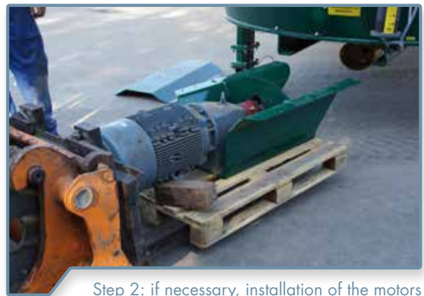
Step 2: if necessary, installation of the motors that have been taken over
